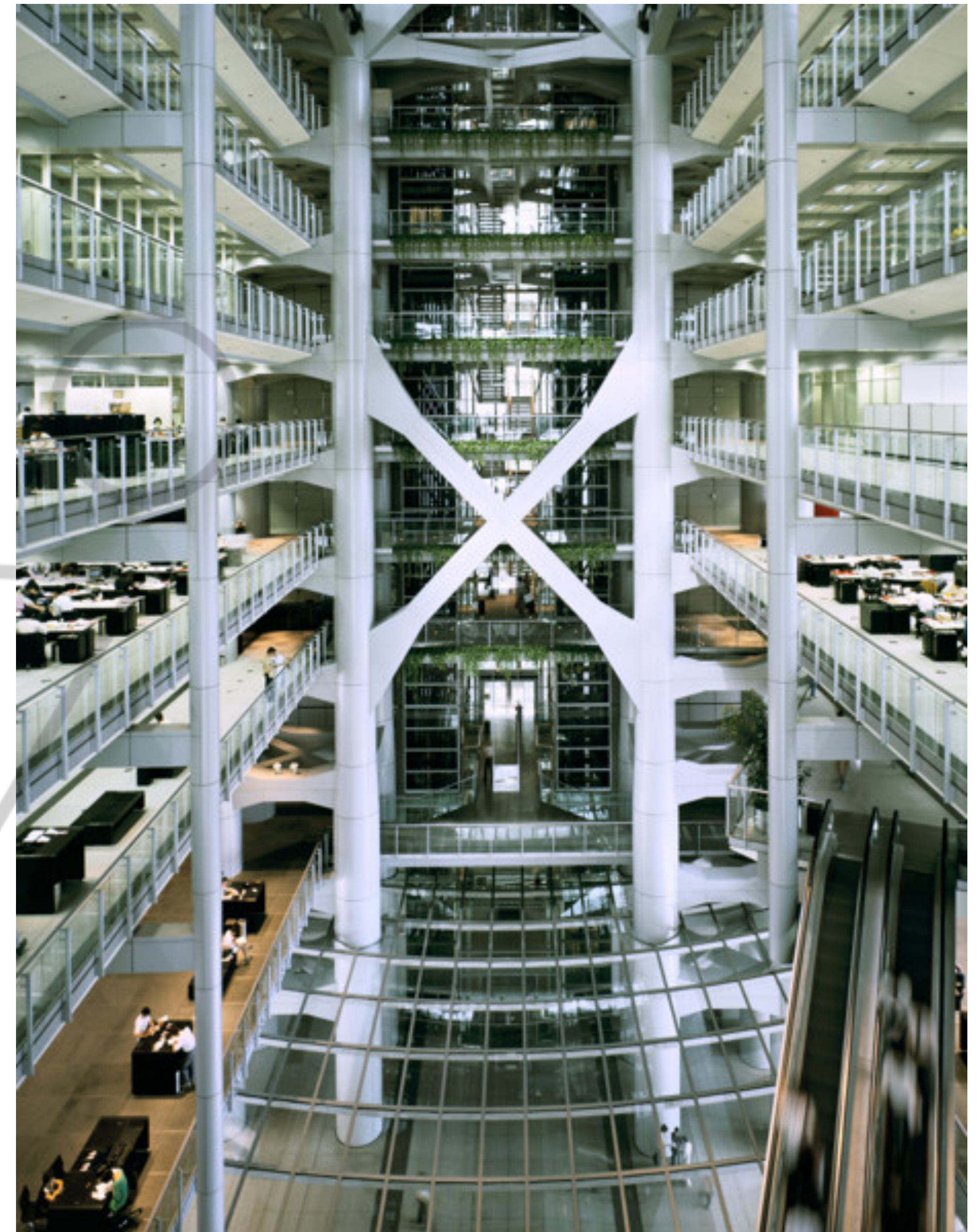
Norman Foster / Ove Arup & Partners, Hong Kong-Shanghai Bank, 1985
