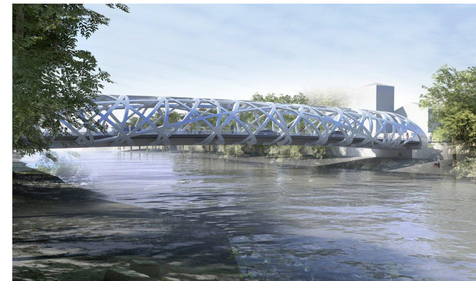
Hans Wilsdorf bridge - Genève, Switzerland - SCIA
