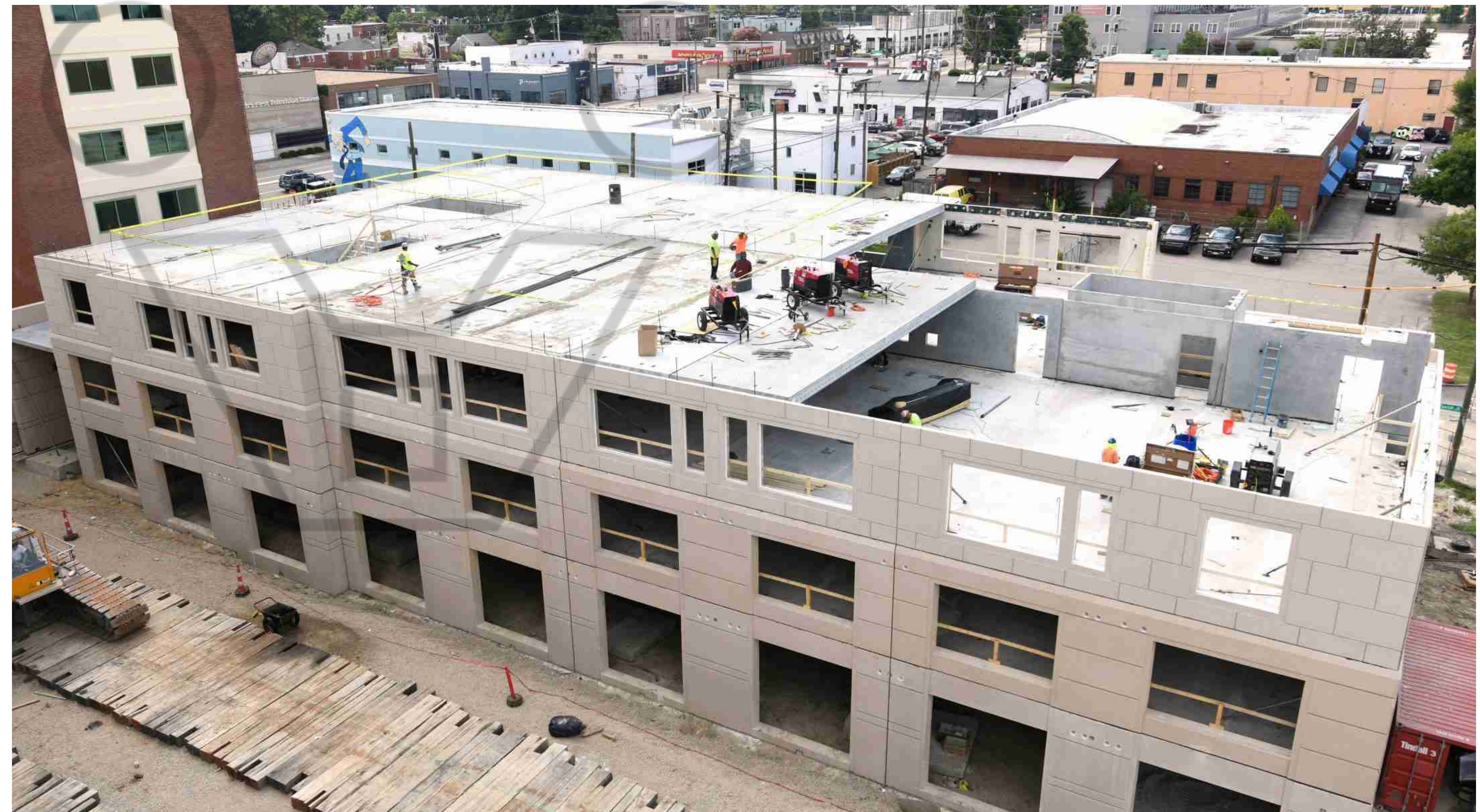
Construction System based on Precast Slab
