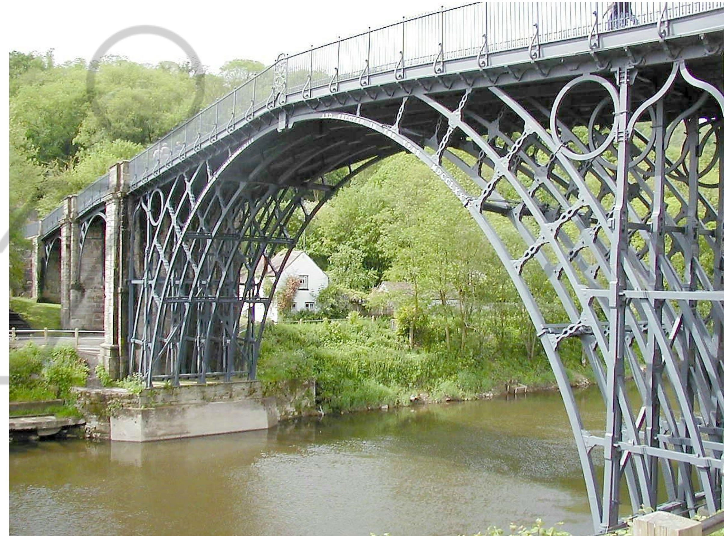
Bridge on River Severn by Abraham Darby III, 1779. A clear example of weaving and how, without scientific knowledge, designer applied the rules of thumbs from other technologies: in this case from the construction of stone arches since cast iron has the same structural behavior of stone.
